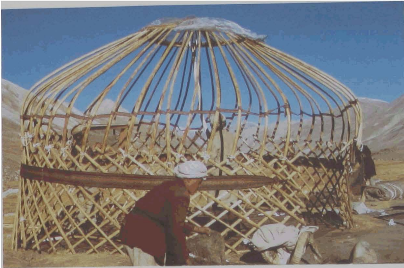
The framework of our yurt being assembled for our occupancy. Covering with yak hair felt squares to make it wind and snow proof, completes its erection. Photo by Edward F. Noack
